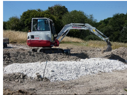
Bee-bank construction work
