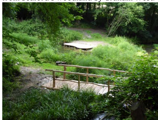
A new bridge and dipping platform
