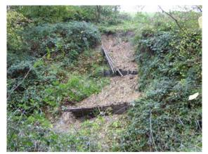
• Heavy rain causes revetment collapse; more work is needed to stop the erosion of the bank.
