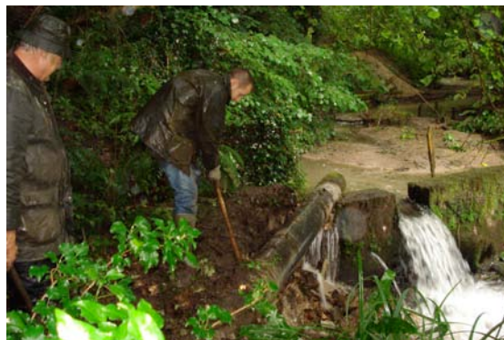
Taking out the pipes
