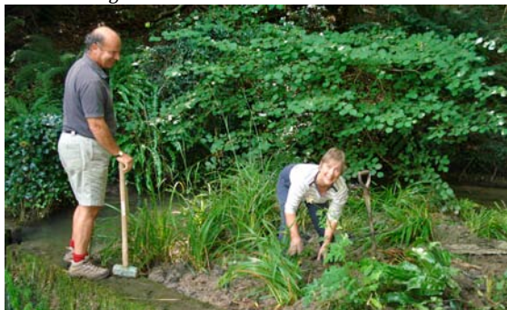
planting up the silt barrier
