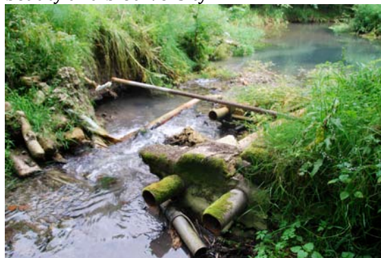
Collapsed old fish farm dams
