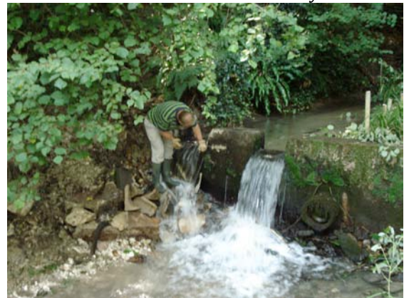
The concrete dam; Robin Bray's first efforts with a hammer and chisel
