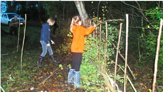
Putting in the binders to the framework of the hedge
