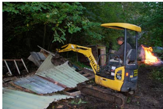
Clearing huts with the digger
